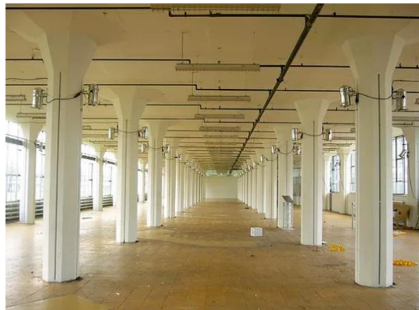
Figure 6. Van Nelle Factory flooring before renovation [30]
