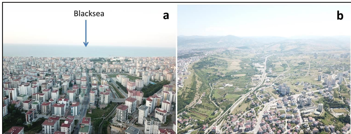
Figure 3: a) The part of the Atakum campus built on the coastal plain. Multi-storey buildings are constructed on alluvial soil. b) Plateau areas. These areas are composed of volcanic-sedimentary soils and are more durable.
