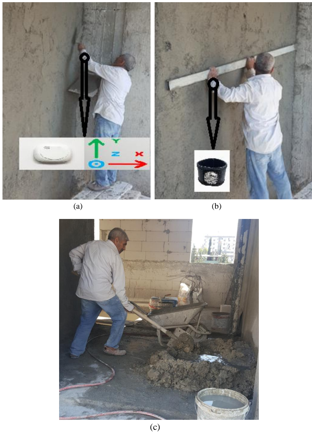
Figure 1. Construction Roughcasting Activities (a) Roughcasting activity with sensor detail, (b) Lining Activity with wrist band and (c) Material Preparation Activity
