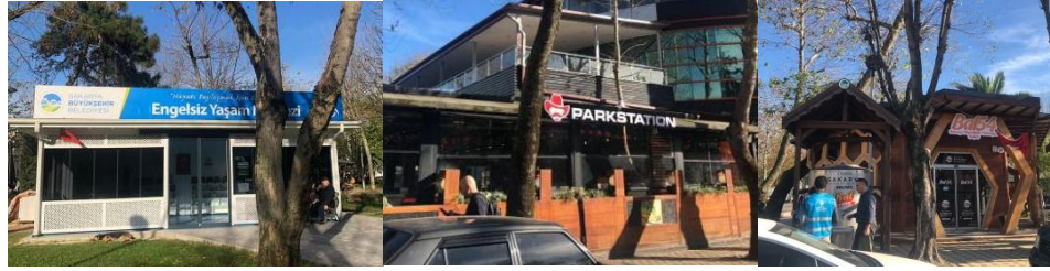
Figure 4. Views around the study area (Barrier-Free Living Centre, BELPAŞ and sales units) (Authors)
