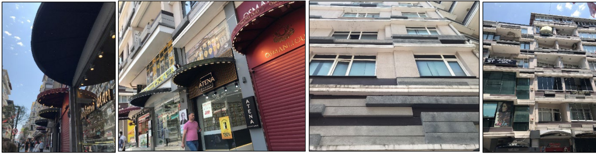
Figure 9 Street frontage after improvement; awnings added to building and shop entrances (photo: documented by the authors)
