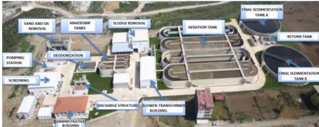
Figure 1. Bird's eye view of Durugöl Sewage Treatment Plant
