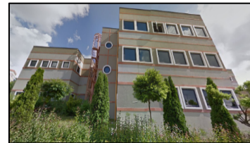
Güney Cephe (Google Earth)
