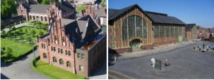
Figure 3 (left). The building designed in Jugendstil by Paul Knobbe. (D. Kaçar Archive)
