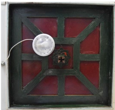
Figure 14. Ceiling Medallion in the Former Exterior Sofa Area of the Mustafa Balcı House
