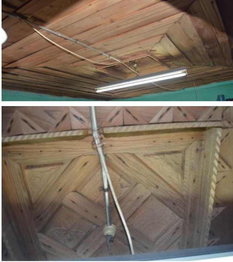
Figure 19. Ceiling and Medallion in the Southwest Room of the Ramazan Genek (Topal) House
