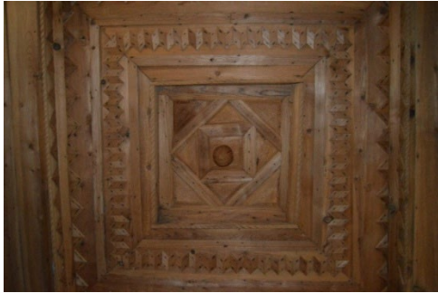
Figure 1 Ceiling Medallion of the Room in the Celal Ayaz House
