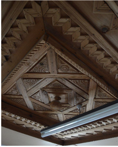
Figure 6. Ceiling of the Room in the Muhammed (Mehmet) Ayaz House
