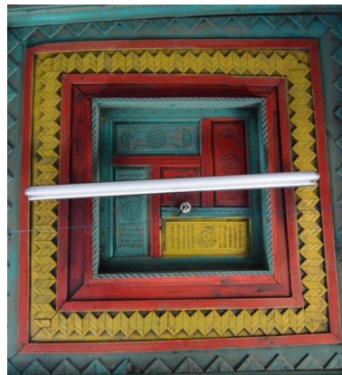
Figure 12. Ceiling Medallion of the Room in the Necip Ayaz House
