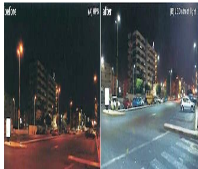
Fig. 1. Night time lighting view of the HPS and LED lamp of different rating
