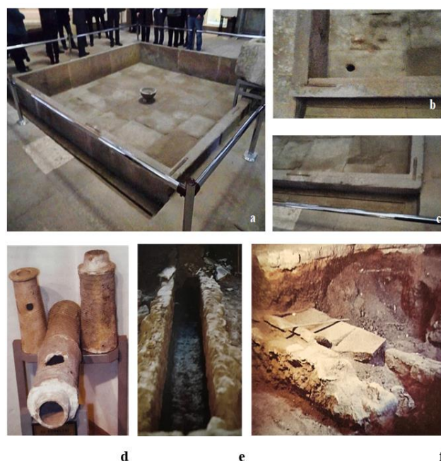
Figure 9. The pool, water channel, and drainage hole of Ince Minareli Madrasa (Author,2026), d- Terracotta pipes of the subsurface canal network of the Ince Minareli Madrasa [29], e,f- open canal [30]
