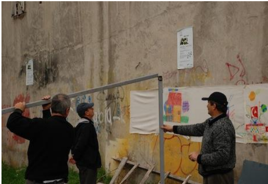
Figure 13. Dismantling the houses (Özdamar, 2010a)
