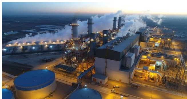
Figure 1. Bismayah 4500 MW combined cycle power facility.
