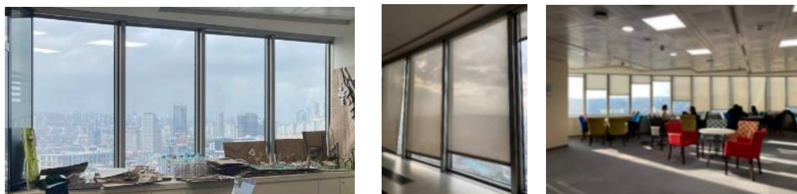
Figure 2: The left side features an interior view of the curtain glass facade utilized in the project on the 18th floor. In the center and to the left, roller blinds are employed in the offices. (Photograph by Nahid Babaei)
