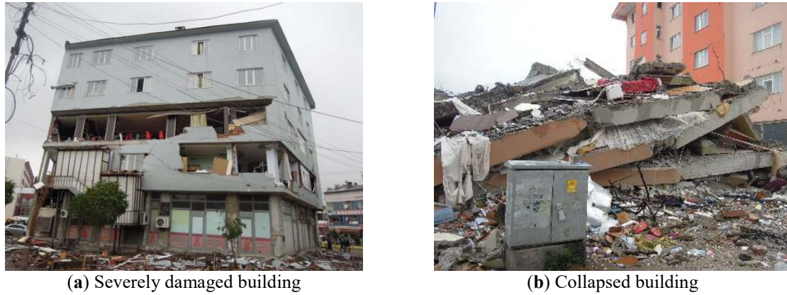
Figure 1. Severely damaged and collapsed buildings in Erciş Town.
