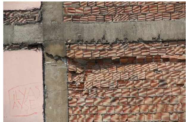
Figure 3. The damaged column (1/2)
