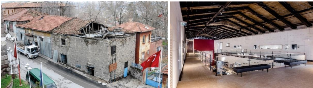
Figure 2. The State of the Building Before Intervention- Interior space [22] [26]
