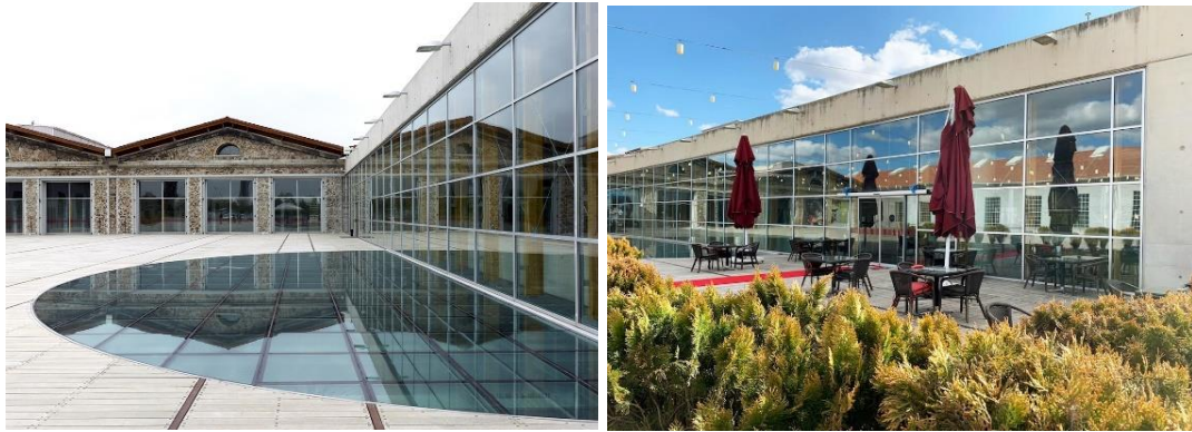
Figure 7. Additional Structure and Hangar [30]
