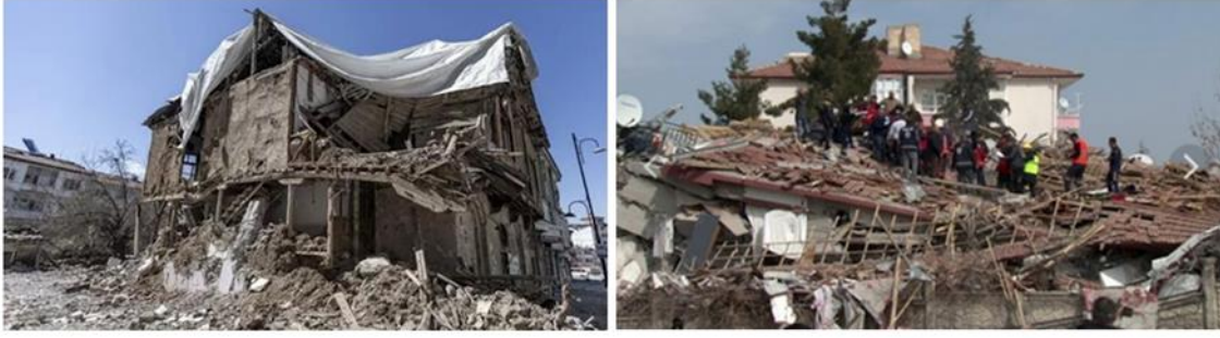
Figure 10. The Impact of the February 6 earthquakes on Malatya (Author's Personal Archive, 2023)
