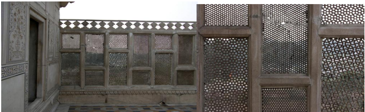
Figure 18. The walls and balcony railings are also carved jalis, with six and 8-point geometrical patterns. (Markcareaga, 2004)
