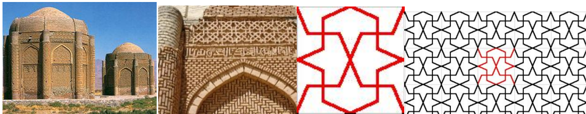
Figure 6. The tomb towers of Kharāqan (right) and the brick wall and arch detail (Zereshk, 2008) The pattern tessellation drawn by authors
