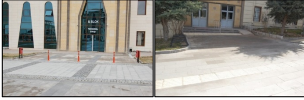
Figure 9. Some buildings have the same floor entries with the floor.
