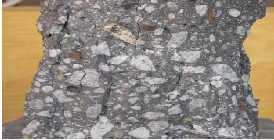
Figure 2: Fracture surface after compressive test
