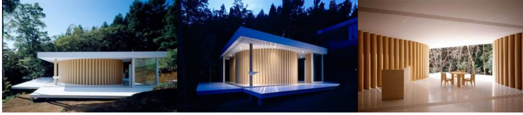
Figure 10. Shigeru Ban's Paper House (1995), residential project using cardboard tubes as structural elements, reflecting sustainability and the traditional Japanese concepts of impermanence and naturalness. [21].
