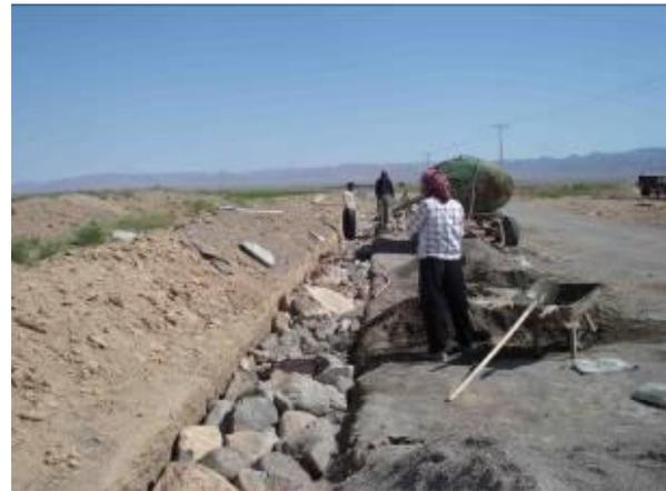
**Figure 12.** Utilizing locally materials and workers and (LBT) in establishing infrastructures for rural roads in a disadvantaged region in South Khorasan province (By author, Sep 2010).
