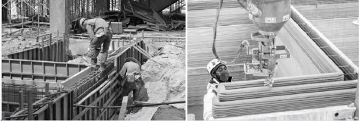
Figure 9. Construction process with conventional method and construction method with 3D printer [2]
