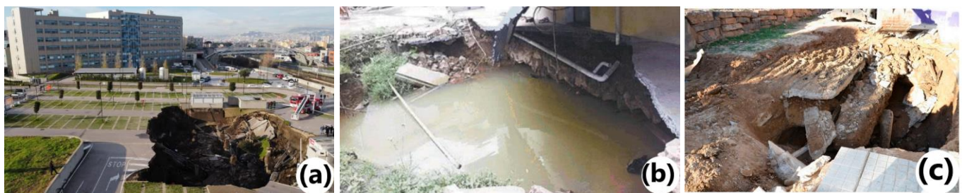
Figure 9. Sudden Collapses and Surface Settlements Caused by Changes in the Groundwater Level and Heavy Rainfall a. Italy b. China c. Spain
