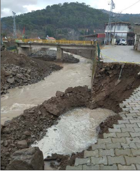
Őekil 11: Karadere Kırsal Mahallesi yapay kanalda oluŐan zarar / Figure 11: Damage occurring in the artificial channel in Karadere Rural Neighborhood (16.01.2024).
