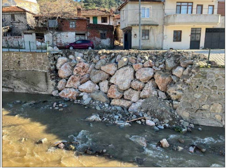
Őekil 12: Karadere Kırsal Mahallesi yapay kanalın onarılmıŐ halinin g r nt s  / Figure 12: The view of the repaired artificial channel in Karadere Rural Neighborhood (23.01.2024).
