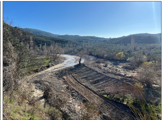
Őekil 14: Akarsuyun taŐkın anında yatak deđiŐtirerek  arpak noktasını aŐındırdıđı nokta ve DSI'nin demonstrasyon  alıŐması / Figure 14: The point where the stream changes its channel during a flood and erodes the impact point, and the demonstration study conducted by the General Directorate of State Hydraulic Works (DSI) (23.01.2024).
