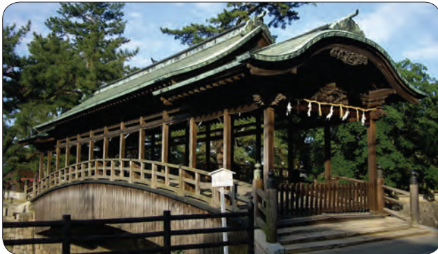
Fotoğraf 35 - Japonya’da geleneksel ahşap bir köprü / Traditional wooden bridge in Japan. (Saya-bridge in Kotohira, Kagawa prefecture, Japan) https://commons.wikimedia.org/wiki/Category:Saya-bridge,_Kotohira#/media/File:Saya-bridge01.jpg
