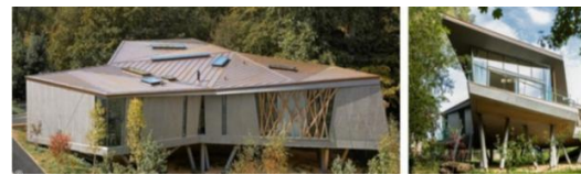
Figure 2. Exterior view of the Oxford Maggie's Centre [29].
