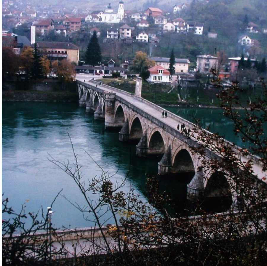
Figure 1: Drina Bridge (UNESCO).
