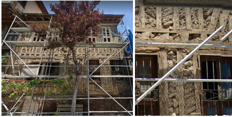
Figure 6. Adobe filling between timber frame (URL-1)
