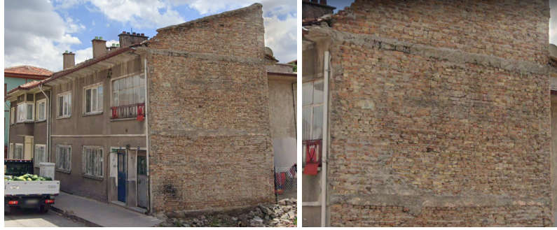
Figure 8. Brick masonry house, reinforced concrete floor (URL-1)
