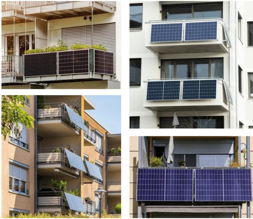
Figure 1. Examples of balcony plug-and-play PV systems.
