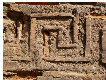
Figure 9 Greek key meander executed in the brick, south facade of the Christ Pantepoptes Church/ Eski Imaret Cami, photo: ©Jasmina S. Ćirić.
