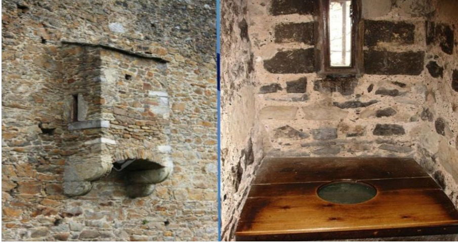
Figure 3: The Image Shows Both The Interior And Exterior Views Of a Garderobe-A Type Of Toilet Built As A Protruding Structure in a Medieval Castle (Cartwright, 2018).
