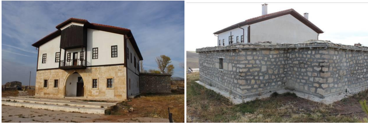
Figure 1. General View of Mihrali Bey Mansion
