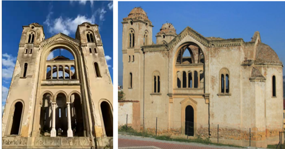
Figure 4. Western and southern façade views of the church.
