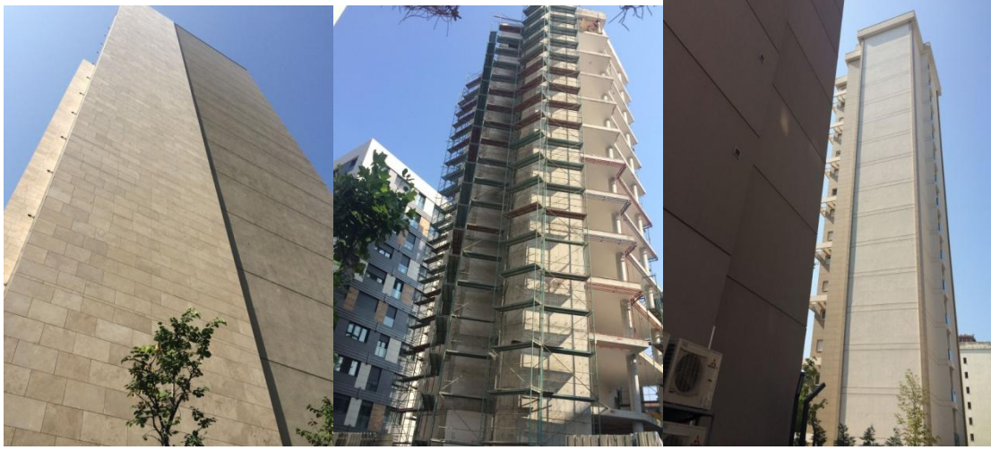
Figure 3a. Sample building 3 and facades of newly constructed adjacent buildings. Figure 3b. Sample building 8 & 9.
