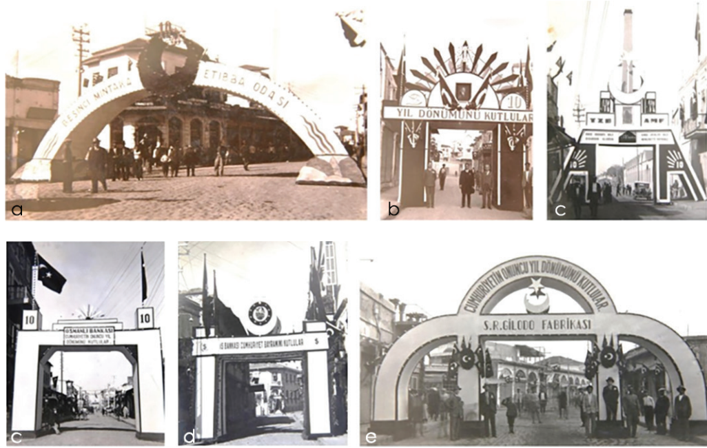
Figure 5. a) Tak of the Chamber of Physicians, b) Tak of Ziraat Bank, c) Tak of Salonika Bank, d) Tak of Ottoman Bank, e) Tak of İş Bank, f) Tak of S.R. Gileto Factory (Kalafat & Kalafat, 2022)- Adana, 1933.
