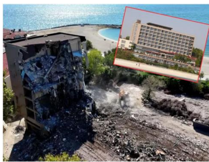
Figure 7. The Demolition of Yesilköy Çınar Hotel, İstanbul (Gzt, 2025)
