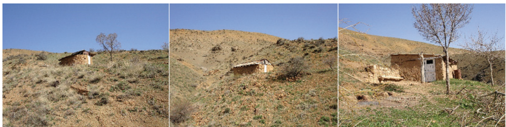
Figure 6. View of the three structures within the Seyids Pir Complex (author's archive).
