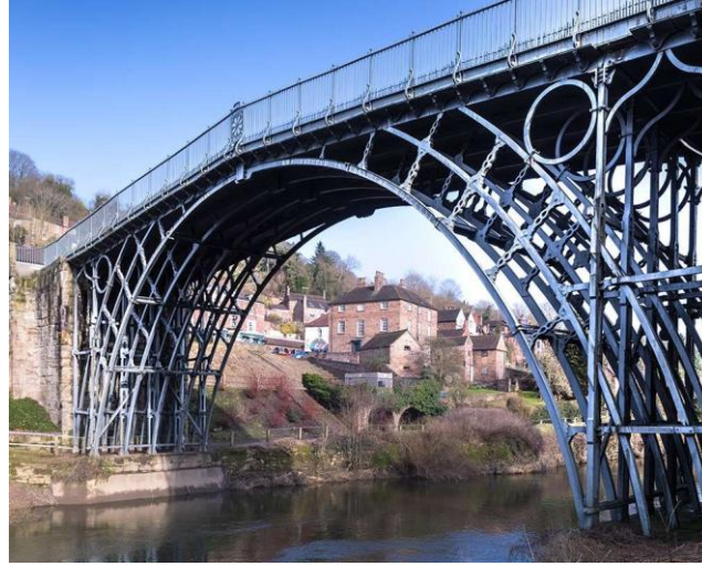
Şekil 3. Coalbrookdale Iron Bridge (URL 3)
