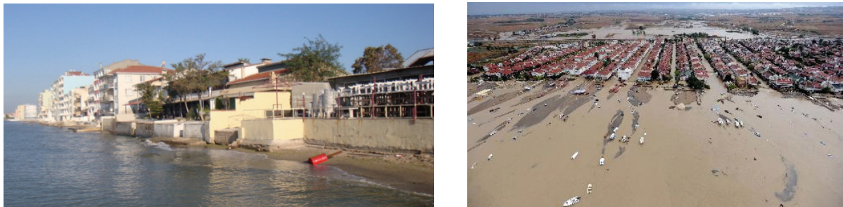
Figure 10. Buildings on the shoreline prevent surface runoff from the catchment area into the Marmara Sea (Marmara Sea coast of Istanbul, September 9, 2009).
