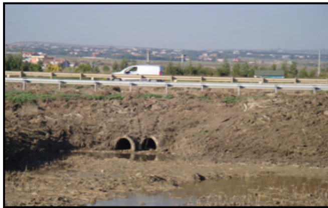
Figure 7. Filling under D 100 Motorway in Tuzla valley bottom and pipe culverts.
