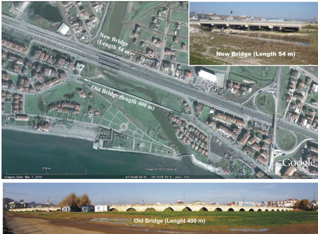
Figure 9. There are two bridges in the same location on the D100 motorway. The older one was built by Mimar Sinan c. 1560. The second bridge was constructed in the last decade.
