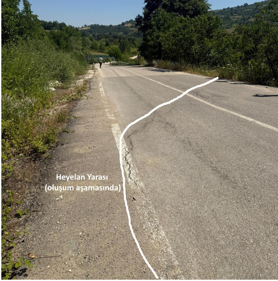
Őekil 13: Muratbey Kırsal Mahallesi ve Hayriye Kırsal Mahallesi Arasındaki Yolda Heyelan Yarası Yeniden Oluřum Ařamasında (28.06.2025) / Figure 13: Landslide scar in the process of reactivation on the road between Muratbey and Hayriye rural neighborhoods.
