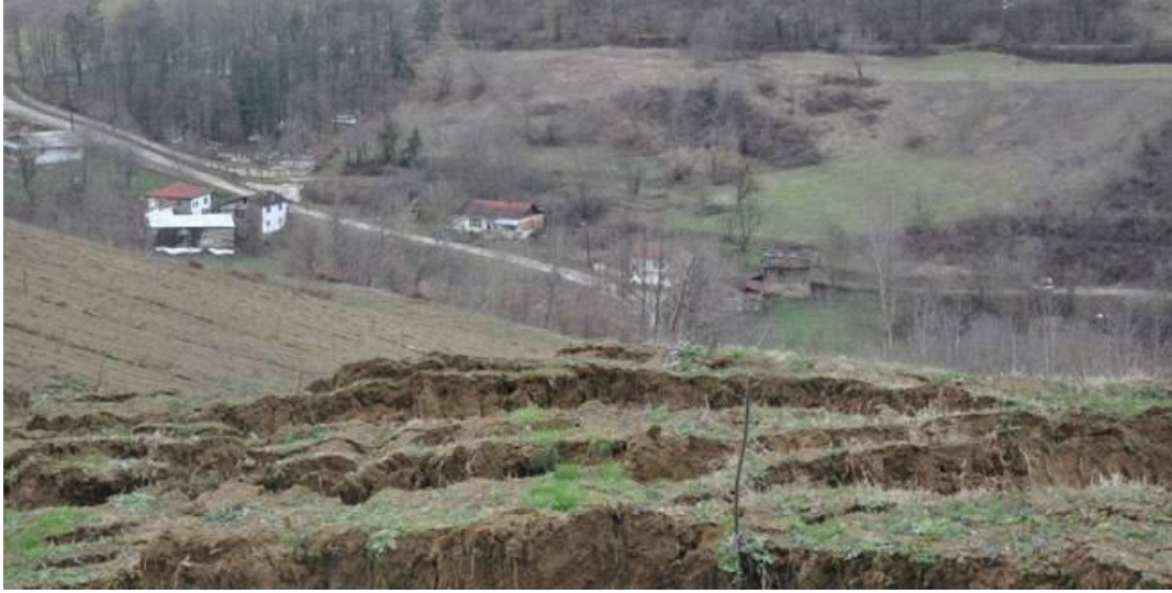
řekil 9: Muratbey Kirsal Mahallesi heyelan alanı kaynak noktasından güneybatı yönlü ekilmiř fotođraf (2015) Kaynak: URL1 / Figure 9: Photograph taken from the source point of the landslide area in Muratbey rural neighborhood, looking southwest (2015). Source: URL1
