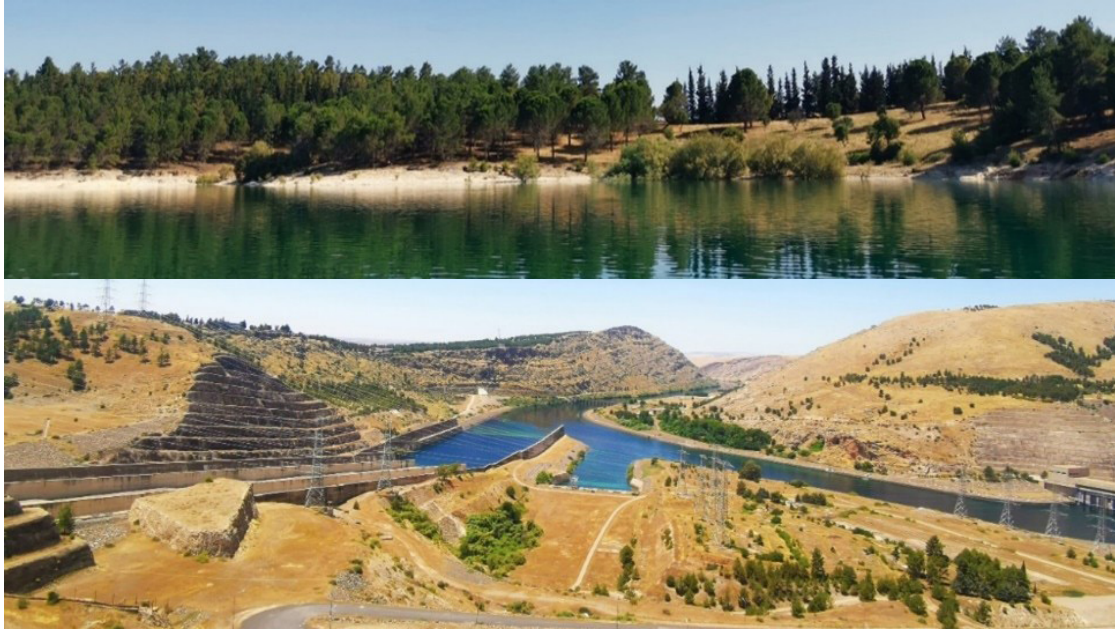
Figure 1. The Atatürk Dam, which meets the major irrigation and energy needs of the GAP Region, and afforestation activities
