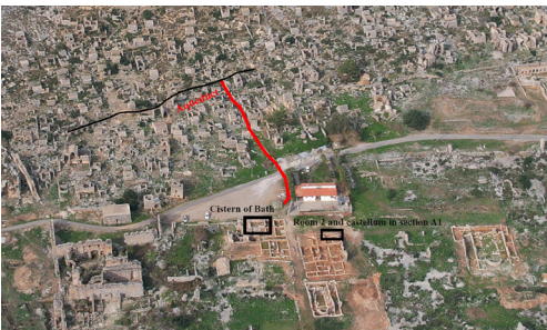
Fig. 8.4. Aerial view of aqueduct line and the possible water supply line connecting the Central Bath and Room 2 of Section A1 of the building.
