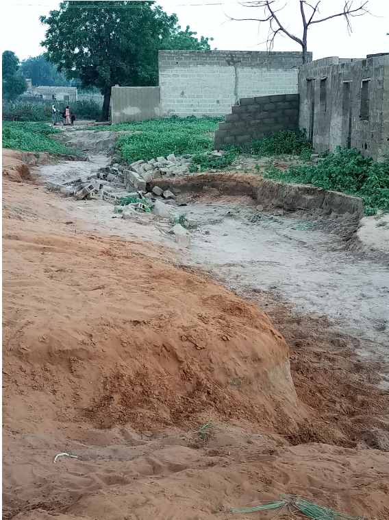
Figure 17: Housing Construction Triggering a Ravine (2021) source: Abdou Sitou L.
