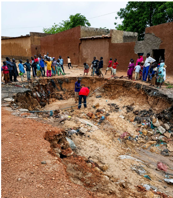
Figure 12: Headcut retreat after a 73 mm rainfall event (42 m 3 of soil removed) source: Abdou Sitou L., 07/09/2021.
