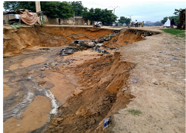
Figure 9: Gully erosion in the N'Wala neighborhood (right side of R3, depth 2.07 m). Figure by Abdou Sitou L. (2020).
