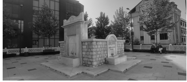
Figure 13. Adile Sultan Namazgah (1886/7), Dudullu. (Source: Author)
