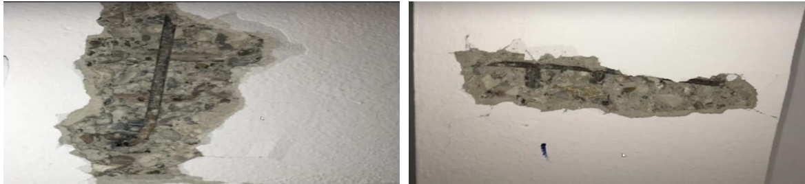
Figure 4. Reinforcement detection and cover removal procedures
