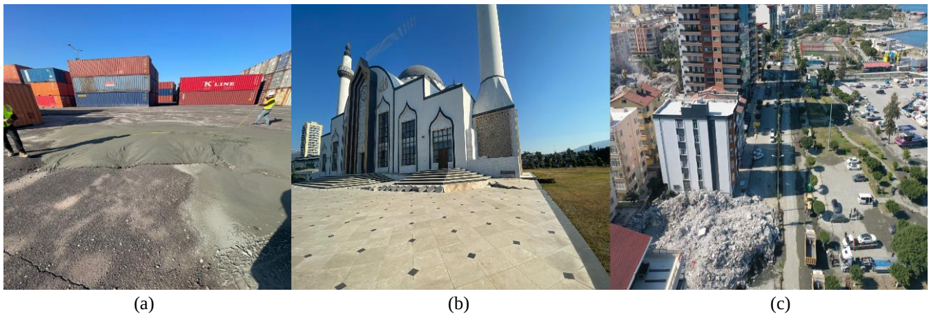
Figure 2. Ground failure observations in İskenderun's coastal fill zone: (a) sand ejecta near the port area, (b) settlement around mosque foundations, and (c) structural collapse and ejecta evidence around Building 3
