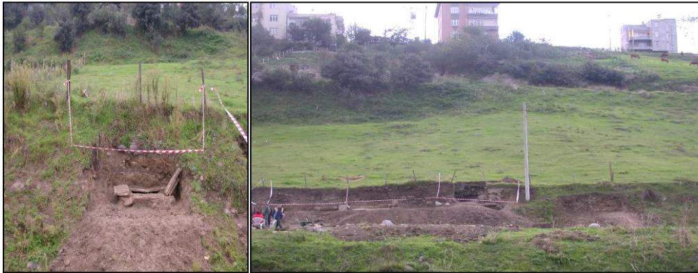
Figure 1: General view of Trial Excavations 1 and 2
