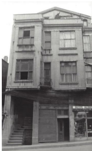
Figure 1. Building from the 80's
