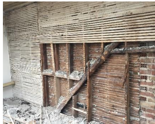
Figure 2. Top floor timber framed wall.
